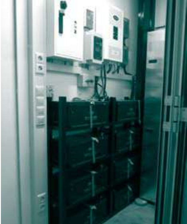
Typical example of an AGM battery bank powering a 3.5kW inverter
